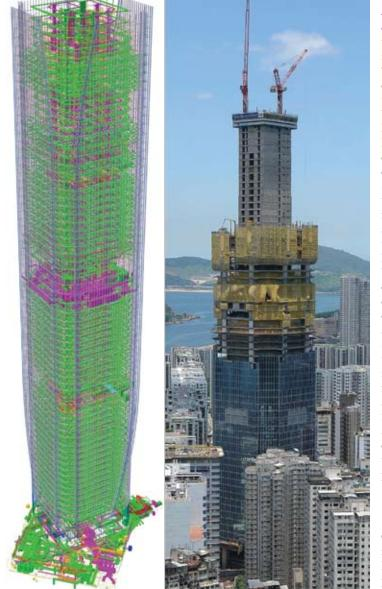
Above: A BIM-generated image of the One Island East project alongside an actual photo in construction. Images courtesy of Gehry Technologies.
